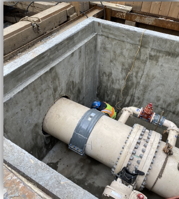
New 36" dia. Butterfly Valve and new chamber under construction at 9 th Ave between W 58 th St & W 59 th St
