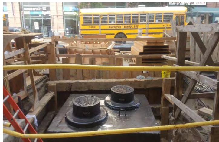
48" Trunk Water Main Regular in Amsterdam Avenue at W.60 th Street
